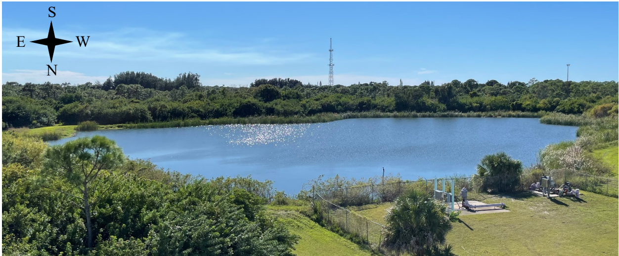
Figure 10: Irrigation Pond and Pumps
